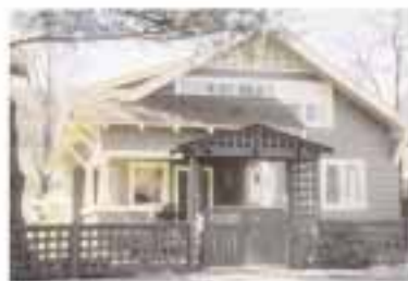
Single planes with exposed structural members and deep overhangs are typical.
