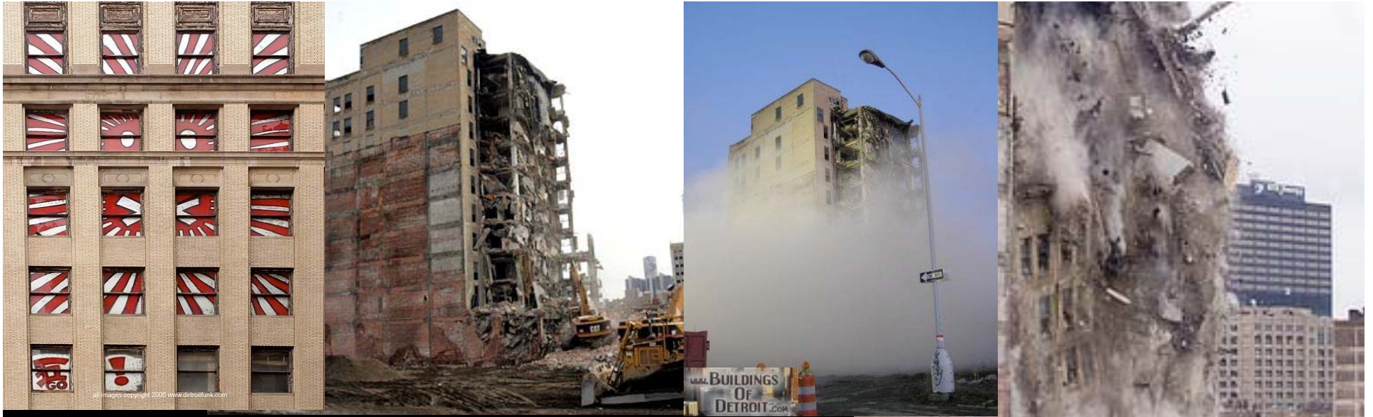
2006 demolition of the Donovan Building - Motown Records Headquarters, 1968 -72
