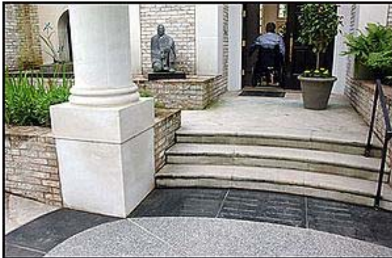
Wheelchair ramp functional, but integrated into design
