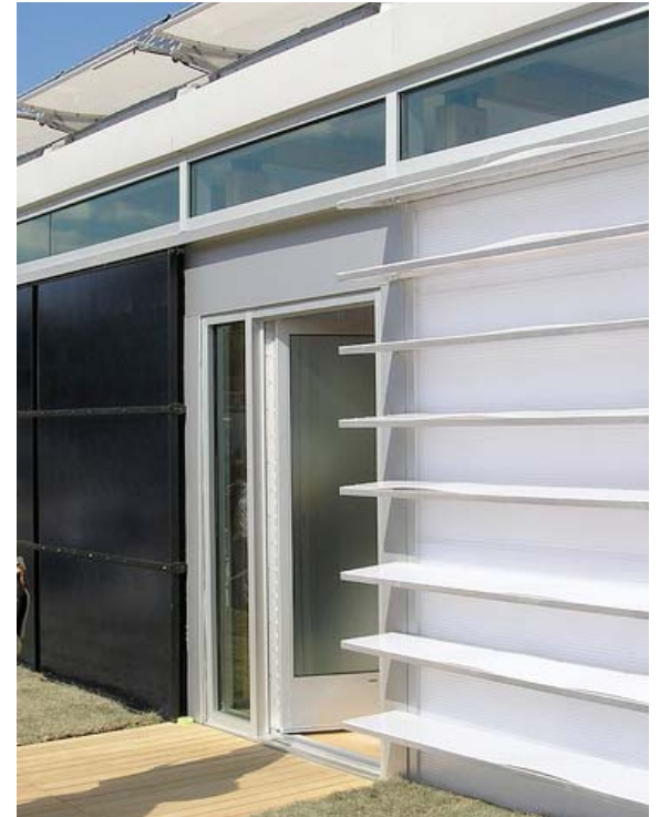
vertical pv rain screen and louvered aerogel walls
