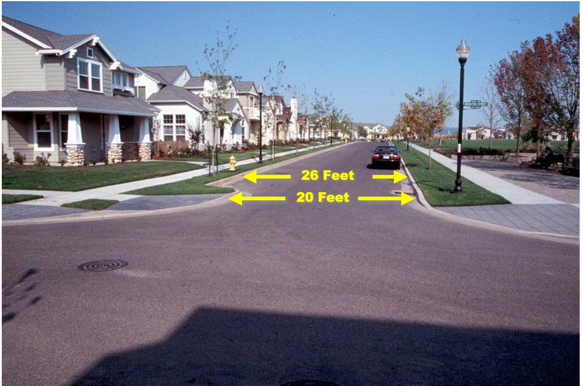
Proper width entry, but protected space is on the wrong side of the intersection
