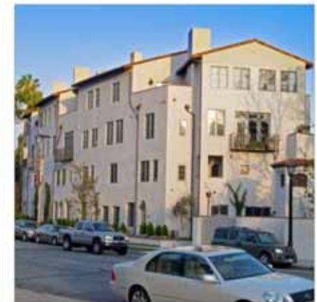
Illustrative Photo: A hybrid court is composed in two parts, a two or three story walk-up attached to a four story point-access building.
