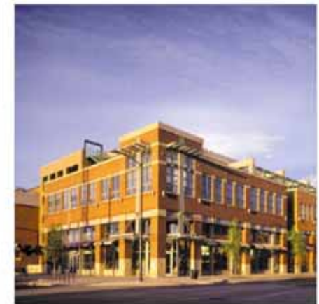
Liner with sheafroof frontage
