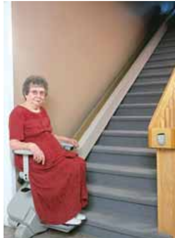
Interior Stair Lift
