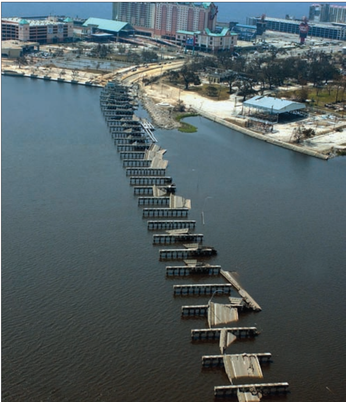
Biloxi-Ocean Springs bridge post-Katrina.
