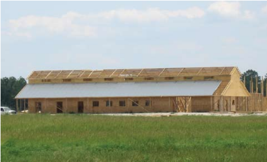
The giant barn/equestrian center at The Oaks includes recycled metal roofing, fiber cement siding, and “green” angle, which is a special high-tech sand that requires less water (to control dust) than natural sand.
