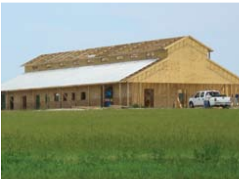
The giant barn/equestrian center at The Oaks includes recycled metal roofing, fiber cement siding, and “green” angle, which is a special high-tech sand that requires less water (to control dust) than natural sand.
