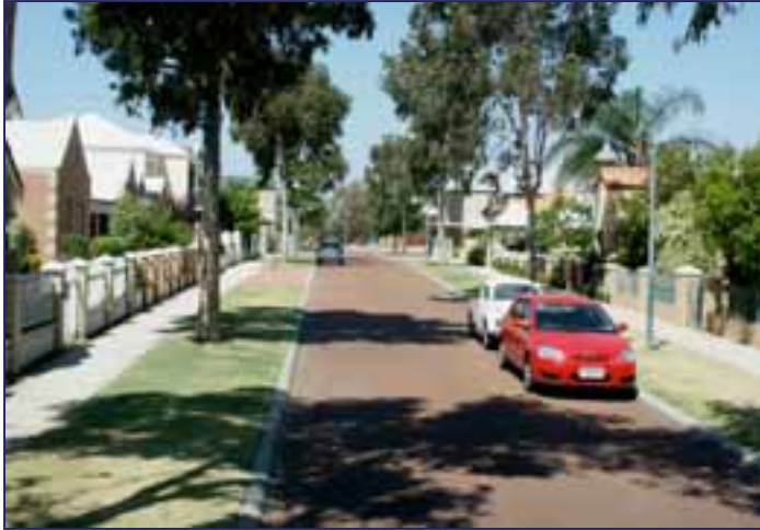
Plaistow St, Joondalup - the first 'demonstration' 6m yield street with footpaths, smaller lots, less front setbacks and rear lane. (Access St D)
