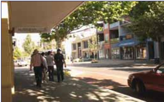
Royal Avenue, Claisebrook - special town centre street. (Integrator B Town Centre without median)
