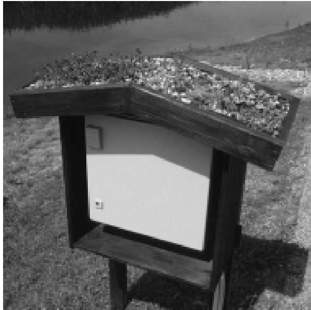
Extensive (green roof)
