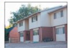
Some newer multi-family structures in Sunnyside are taller and larger than single family or multi-family structures seen traditionally.
