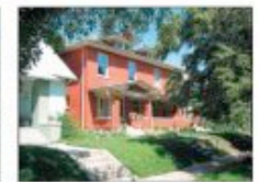
The photograph of a duplex in Congress Park above shows how many traditional multi-family structures fit within the general character of the single-family structures around them.
