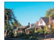
The photograph above shows the variety of roof forms in Sunnyside.
