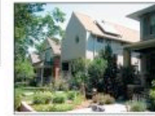
The defining elements of typology A1 are not always recognized in contemporary infill projects.
