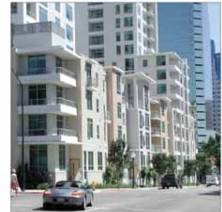
Illustrative Photo: Tower with steep frontages
