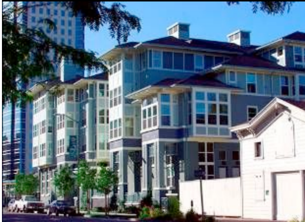
By sinking the garage (one auto per unit) half into the ground below the housing, half-level stoops and porches can line the street edges. This provides life for the street and security to the first level lofts.
