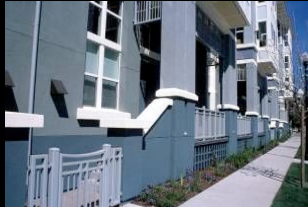
By sinking the garage (one auto per unit) half into the ground below the housing, half-level stoops and porches can line the street edges. This provides life for the street and security to the first level lofts.
