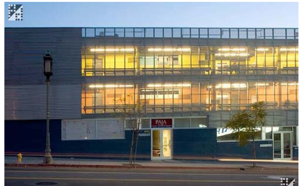
Camino Nueva Charter School , Los Angeles Daly Genik Architects From strip mall to elementary school
