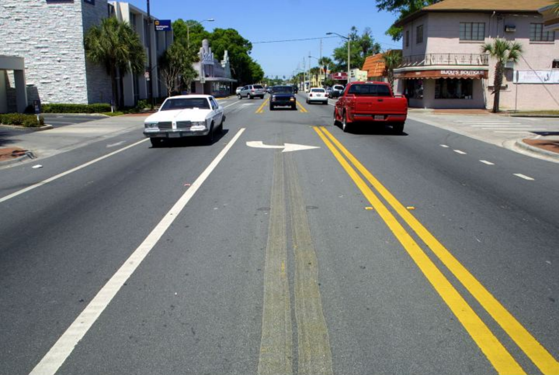
Edgewater Drive, Orlando, Florida 23,000
