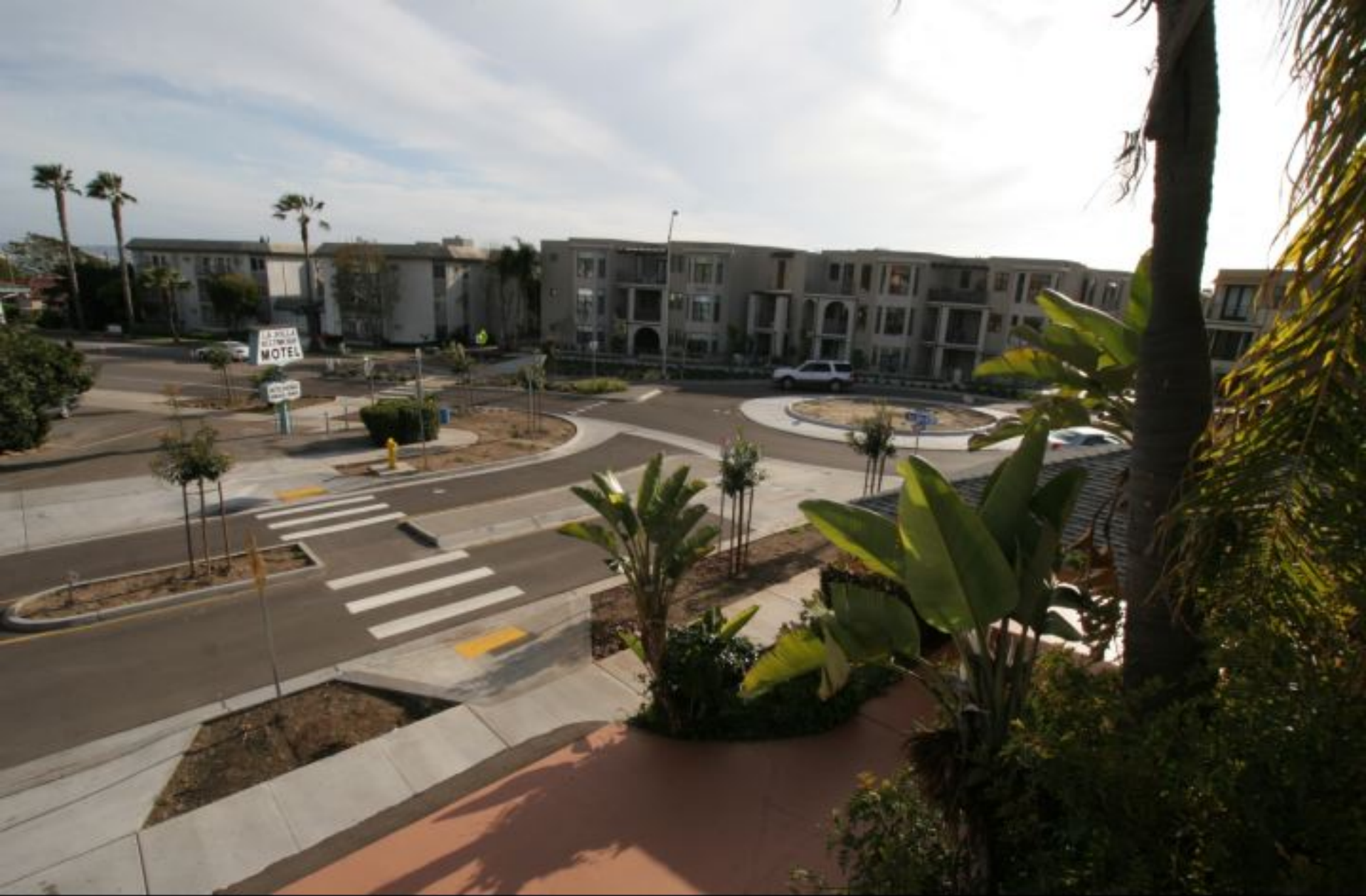
La Jolla Boulevard, Bird Rock, San Diego, California (Five to two lane conversion, after). Four signals and one four-way stop being removed. Back-in Angled parking to be added. (23,000 ADT)
