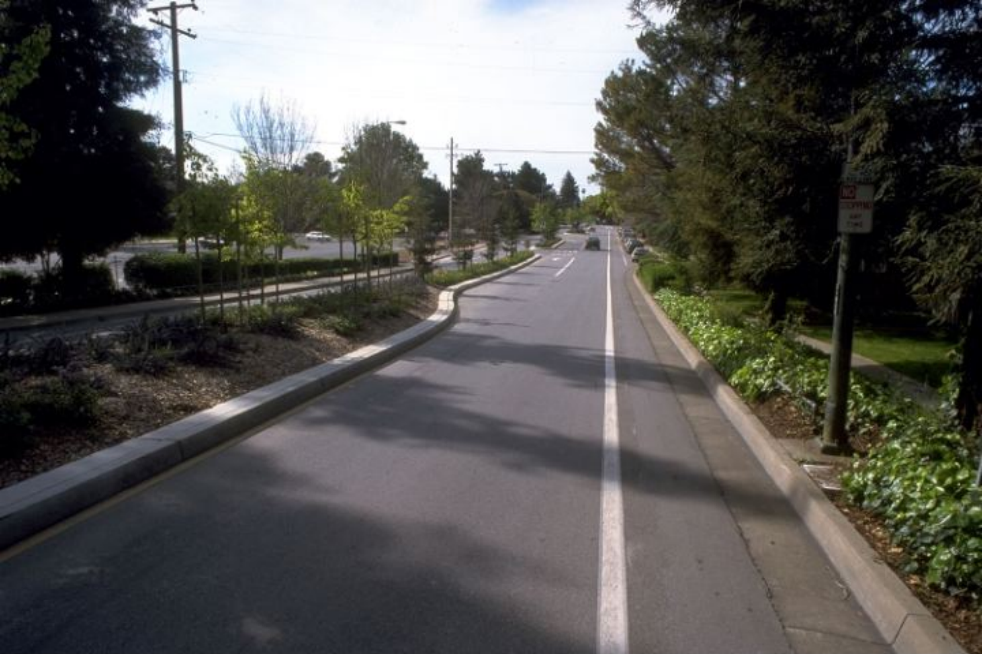
California Street, Mountain View, California
