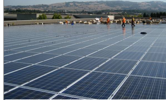
Workers install the solar power plant at Sonoma Mountain Village. The $7.5million plant generates 1.14 megawatts – enough to power 1,000 homes.
