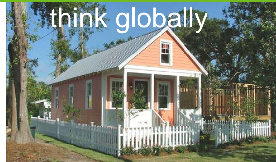
Affordable Katrina Cottage at 510 square feet
