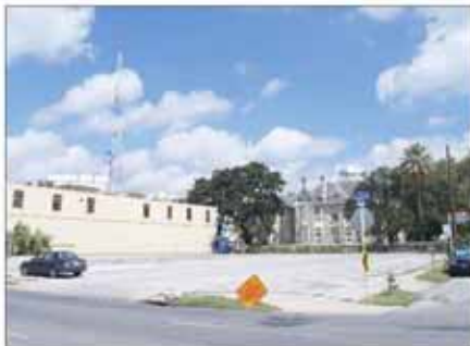
Once Third Street is extended the Municipal Auditorium in the foreground will have a visible presence in the Performing Arts District
