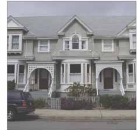
Rowhouse building with front yard and porch frontage
