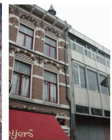
Existing fabric to be restored (Left) and replaced (Right)
