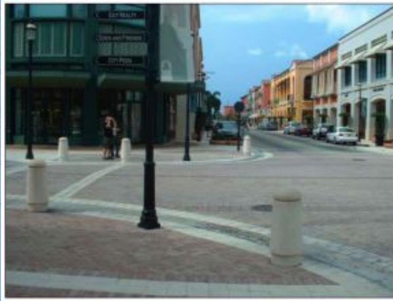
Figure 10.17 Use of contrasting material and bollards to delineate the pedestrian and vehicle areas. Source: Kimley-Horn and Associates Inc.
