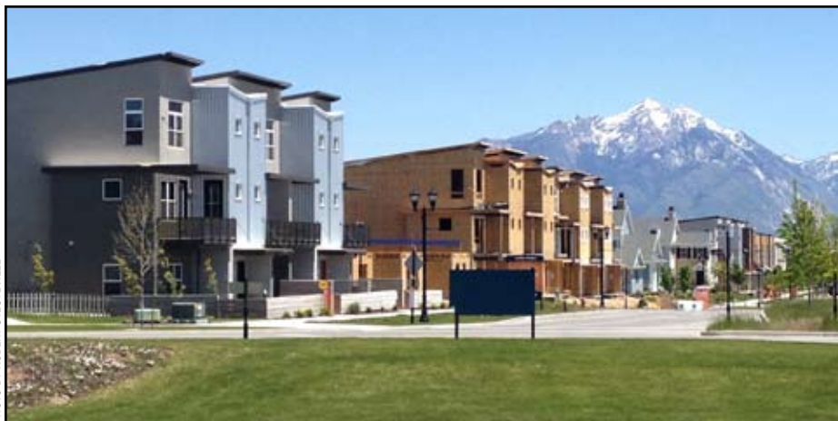
Townhouses built and under construction in Daybreak
