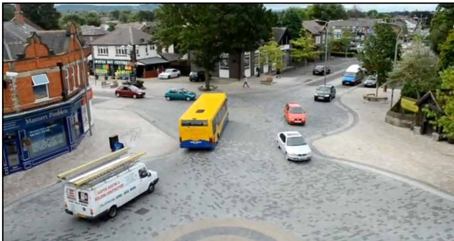
Poynton's 'double roundel' intersection functions as a public space — despite handling 26,000 vehicles per day, including trucks and buses.
