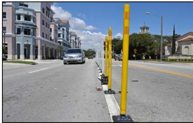
Red Road, Coral Gables, Florida — Plastic sticks are everywhere in modern streets.
