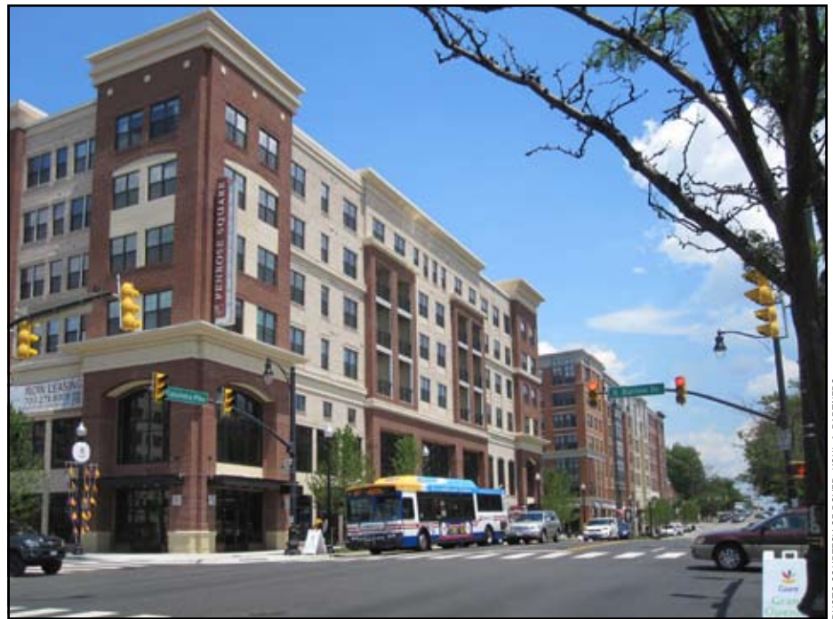
New mixed-use buildings along Columbia Pike in Arlington, Virginia
