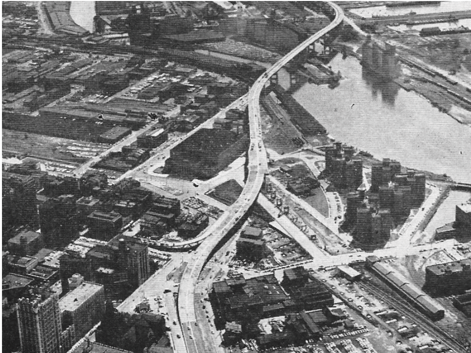
Figure 2: Skyway Bridge recently after construction.
