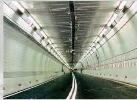
Ted Williams Tunnel - Boston
