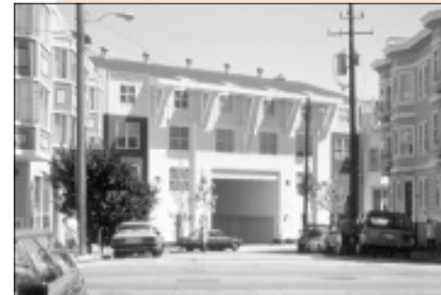
The new building addresses the street and is compatible with its neighbors.
