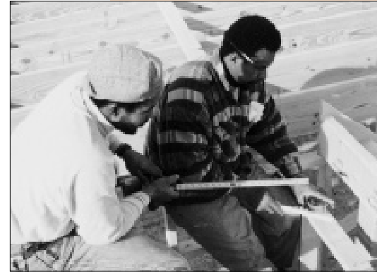
Dixon Construction Company publicly bid their first duplex at $99,999.99 as required to remain under the HUD $100,000.00 minimum performance bonding limit. The duplex was completed with a "Zero" Punch List.
