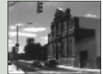
Existing building is to be renovated for new a community center.
