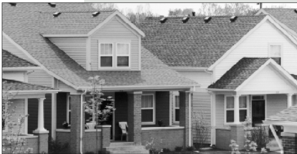
Streetscapes and details from the occupied Concord Village/Eaglecreek HOPE VI development. Residents have taken ownership of their homes, their porches, and their community.
